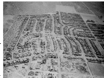
Princess Jeanne Park under construction circa 1955 Courtesy of Pat Boyle
